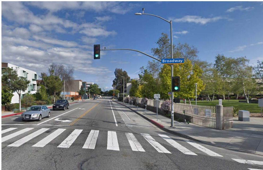
Street view of proposed installation location (looking south on 26 th St)
