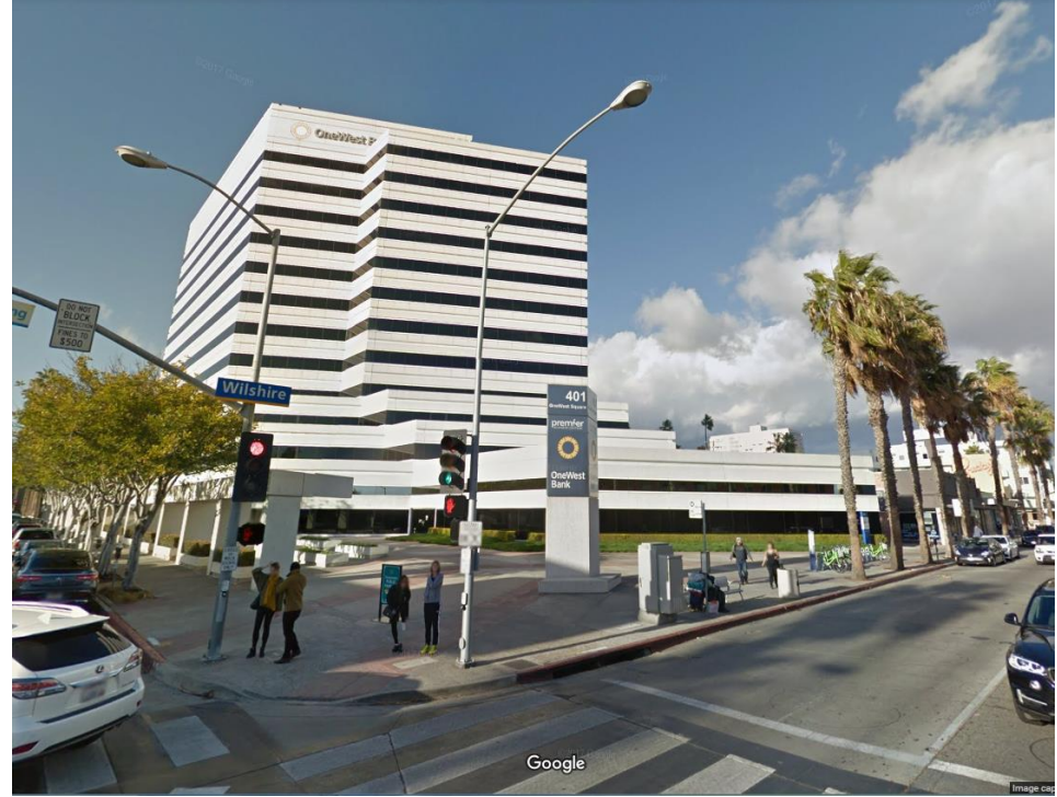
Street view of proposed installation location
