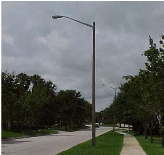
Lighting on Street but not Sidewalks
