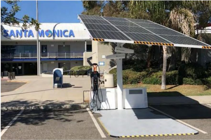
The EV ARC is a solar-powered EV charging station that comes with battery storage, is transportable, self-sustaining, and does not require any construction. The City currently has one of the earlier models located at the Santa Monica Airport. Previous issues of low charge rates in the morning can be mitigated by increasing the battery storage size and/or limiting charging at night.
