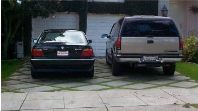
This permeable driveway features concrete pavers.
