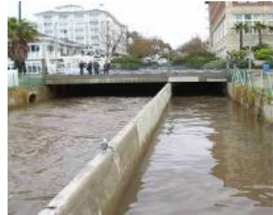
First flush is the phenomenon of the first rain “flushing” out the storm drain system of all the accumulated sediment and trash. The Pico-Kenter storm drain, pictured here in December 2004, is a notorious polluter, draining much of the Westside.
