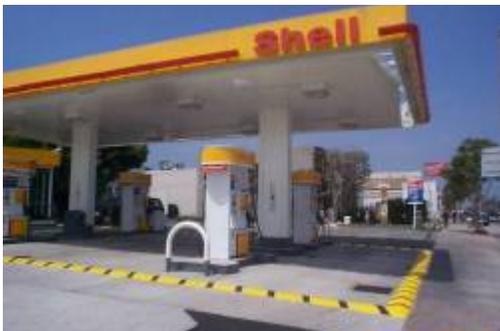
Berm around fueling area to keep any spills or runoff in the fueling area and directed to a catch basin with an insert to remove debris, oil and grease.
