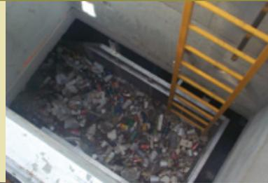
← [Bio Clean Baffle Box™ with floatables, i.e. trash and debris, removed from runoff]
