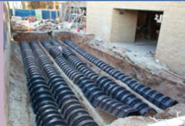
← [Infiltrators® or StormTech® Chambers]
