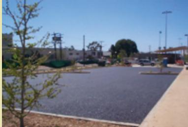
[Permeable Asphalt Parking Lot Absorbing Water] →
