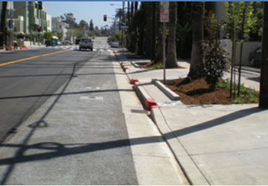
[Depressed Parkway Bioswale and Drip Irrigation] →
