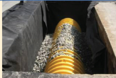
← [Sub-surface Infiltration Basin]
