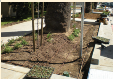
[Depressed Parkway Bioswale and Drip Irrigation] →
